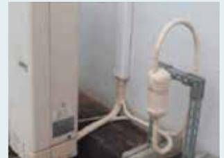
After installation of the device, put thermo-insulator.
